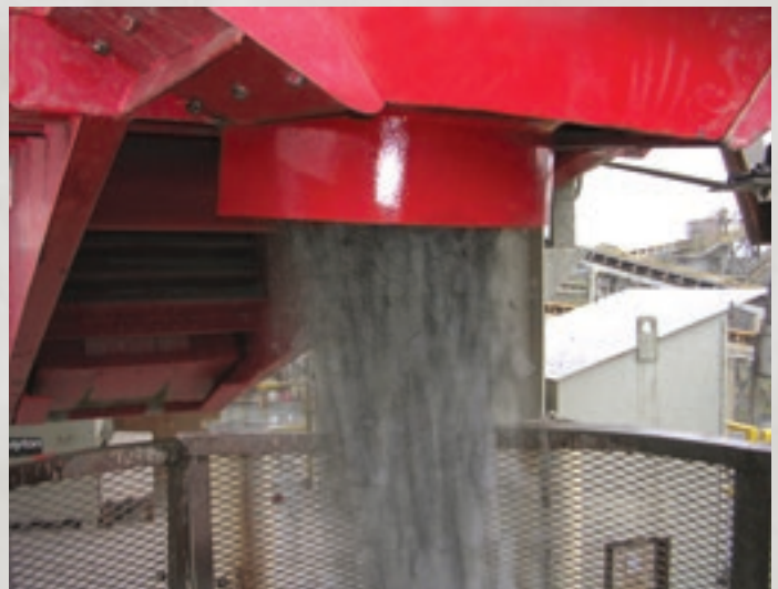
Blended material feeding directly from the Crusher Loading Feeder to the crusher.
